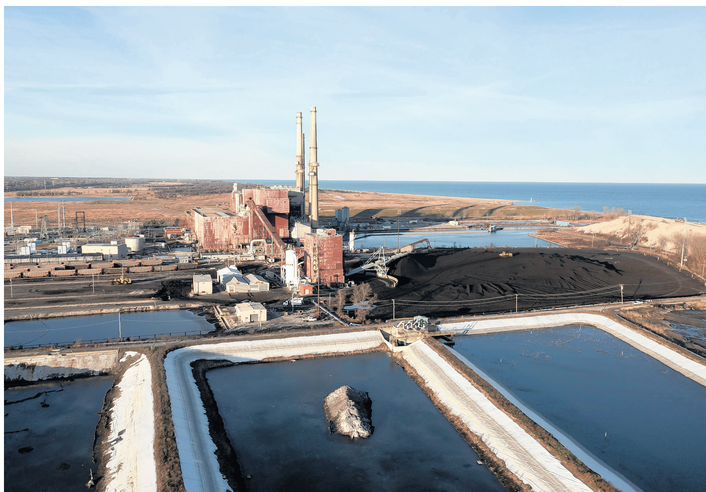
The Waukegan Generating Station coal-fired plant can be seen from North Beach on Tuesday in Waukegan. ERIN HOOLEY/CHICAGO TRIBUNE
