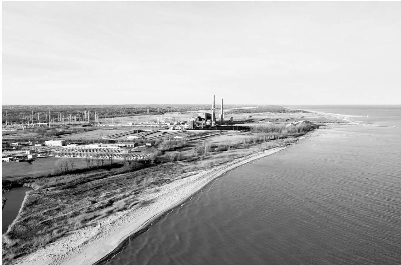
The Waukegan Generating Station coal-fired plant can be seen from North Beach on Tuesday in Waukegan.
